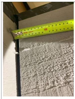
Figure 3 Exterior – Approx 15mm gap between panels at internal corner junction
