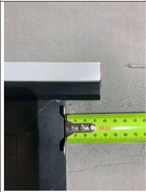
Figure 4 – Head flashing overlap to jamb of only 35mm
