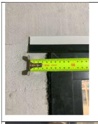
Figure 5 – Head flashing overlap to jamb of approximately 50mm
