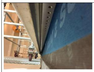
Figure 7 – Sample B, View of cavity closer. Note the Proclima Extasana Adhero.
