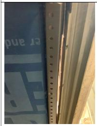
Figure 6 – Sample A, View of cavity closer. Note the Proclima Extasana.
